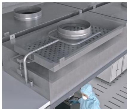
Aerosol Injection Dispersion Ring upstream of the filter
